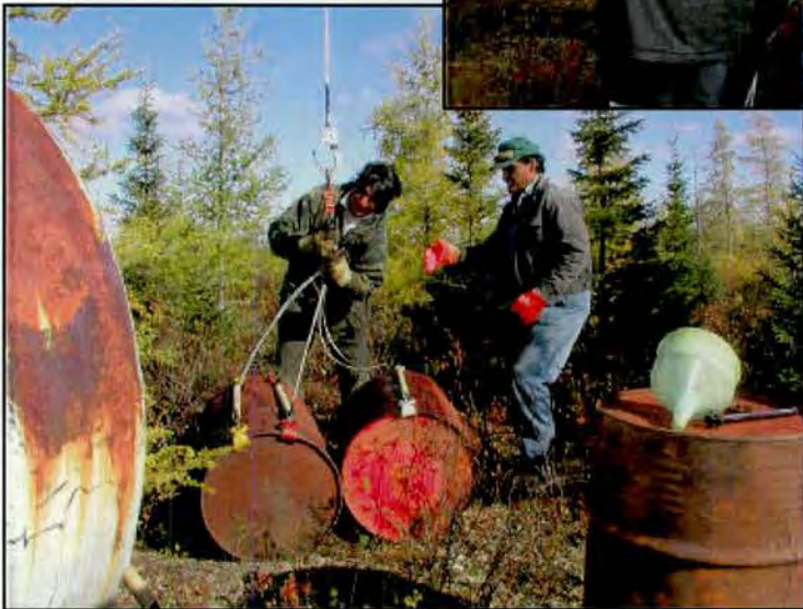
Photo 1 Draining hydrocarbons from fuel tanks into barrels at site 327A and removal of barrels from the site by helicopter (27 September 2002).
