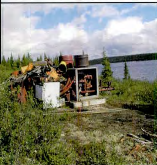
Photo 6 Site 336A: pipeline, hoses and debris near the lake before clean-up work (5 June 2002); worker dismantling the pipeline and debris piled near the pumping station (8 July 2002).
